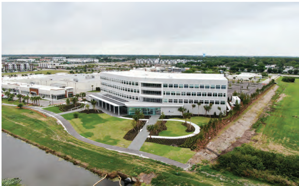
Work on the Sarasota County Administration Center began in late 2023.
